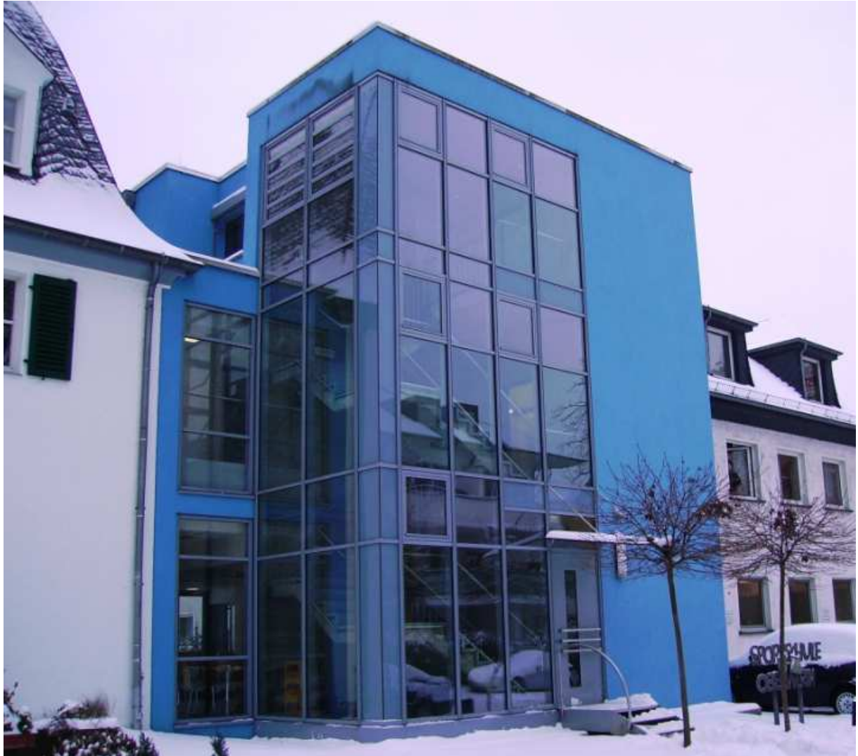
Main entrance Sport Hotel Oberwerth in Koblenz
